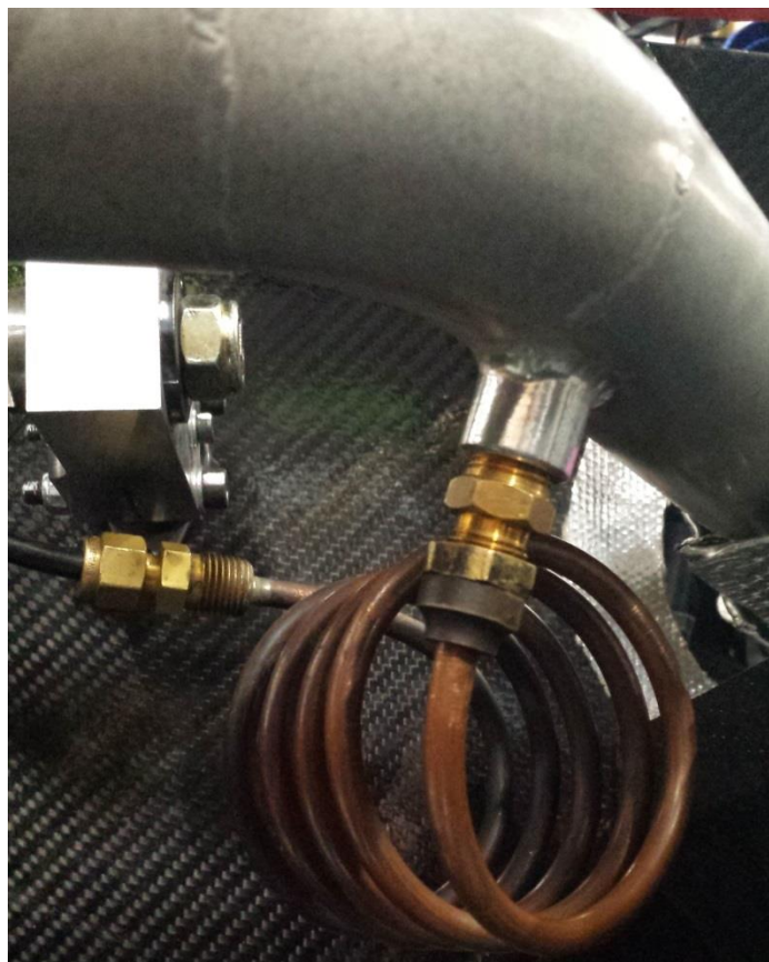
Figure h: The pressure sensor tap tube installed underneath the M19-C's exhaust manifold.
