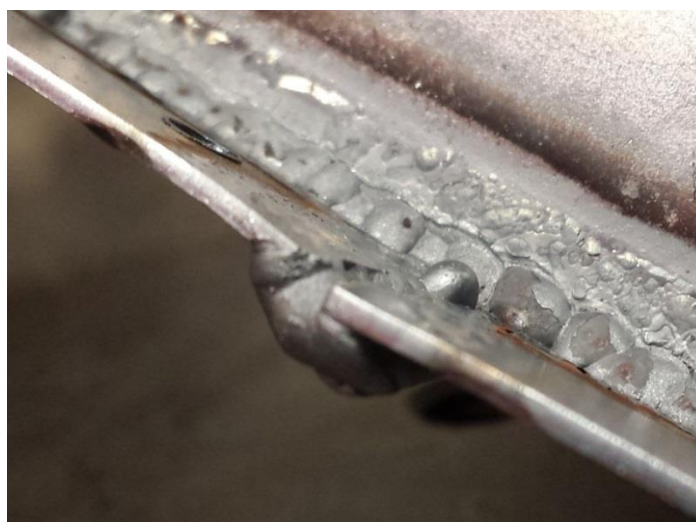
Figure 17: Weld penetration on the underside of the endcap strip. Penetration is undesirable for this particular weld, and the bead near the back had to be removed for the endcap to seal.
